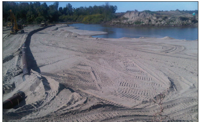
The dredge contractor pumps sand into the scour hole at the center crevasse Friday.
