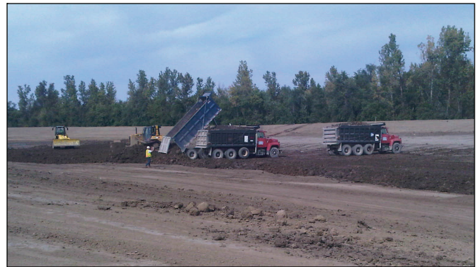
Clay embankment is placed landside of the levee at the upper crevasse Monday to prevent seepage.
